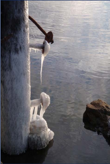
An ice-coated piling
